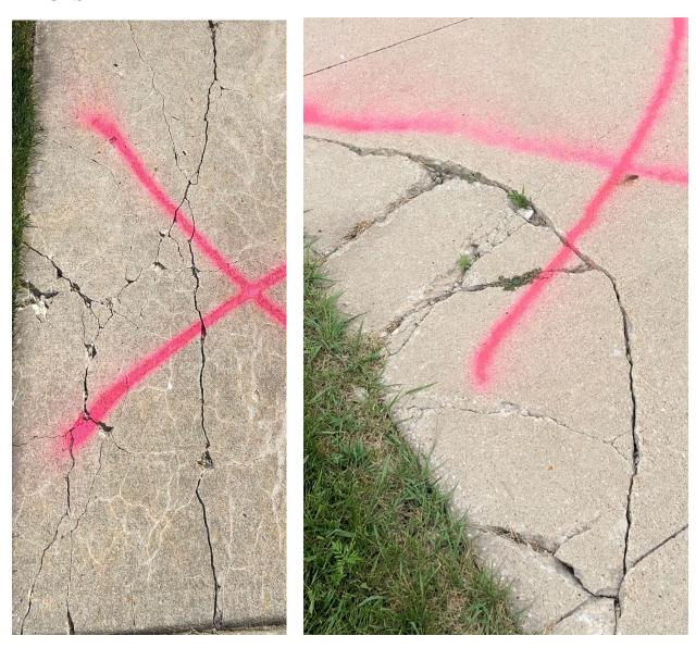
The appropriate repair for this scenario is replacing the panel. Many times this scenario is caused by a vehicle driving over the sidewalk.
