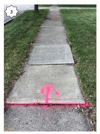
The appropriate repair for this scenario is on a case by case basis, as this condition may be caused by a couple different reasons. If the panel(s) have sunken as in photo (2) you may be able to mud jack or raise the panel(s). If the panel(s) have heaved (raised) as depicted in photos (1&3) then the only repair is to replace the panel(s).
