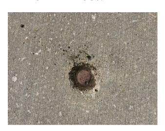
The picture to the left depicts a temporary plug. If you have a temporary plug instead of a service cap please contact the Water Department at 515-967-2454 to get a permanent service cap installed.
