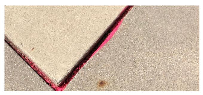
The appropriate repair for this scenario is typically filling in the gap between the two panels. Many times this is caused by deterioration of the expansion joint over time.
