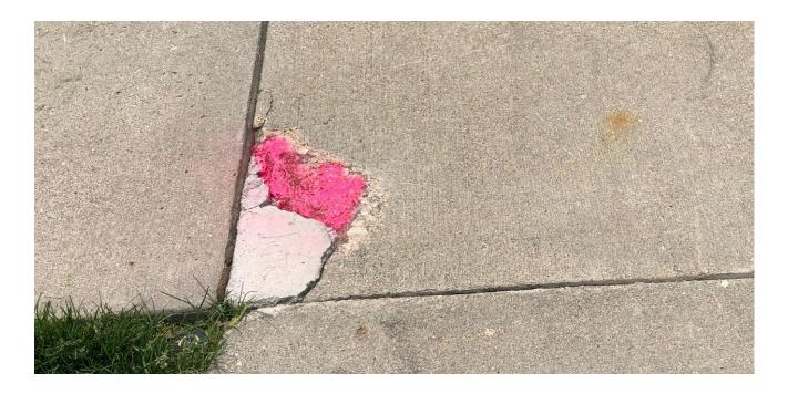
The appropriate repair for this scenario is replacing the panel. Patching or filling in the depression(s) IS NOT an acceptable repair.
