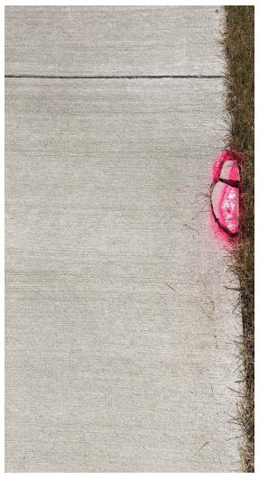
The appropriate repair for this scenario is replacing the panel. If ANY part of the sidewalk is missing in its entirety, Deficiency G applies.
